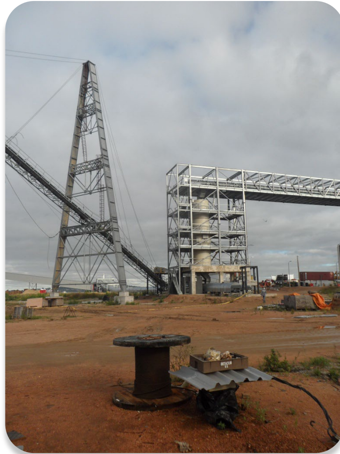
Trapezoidal tie-rod structure for belt conveyors
