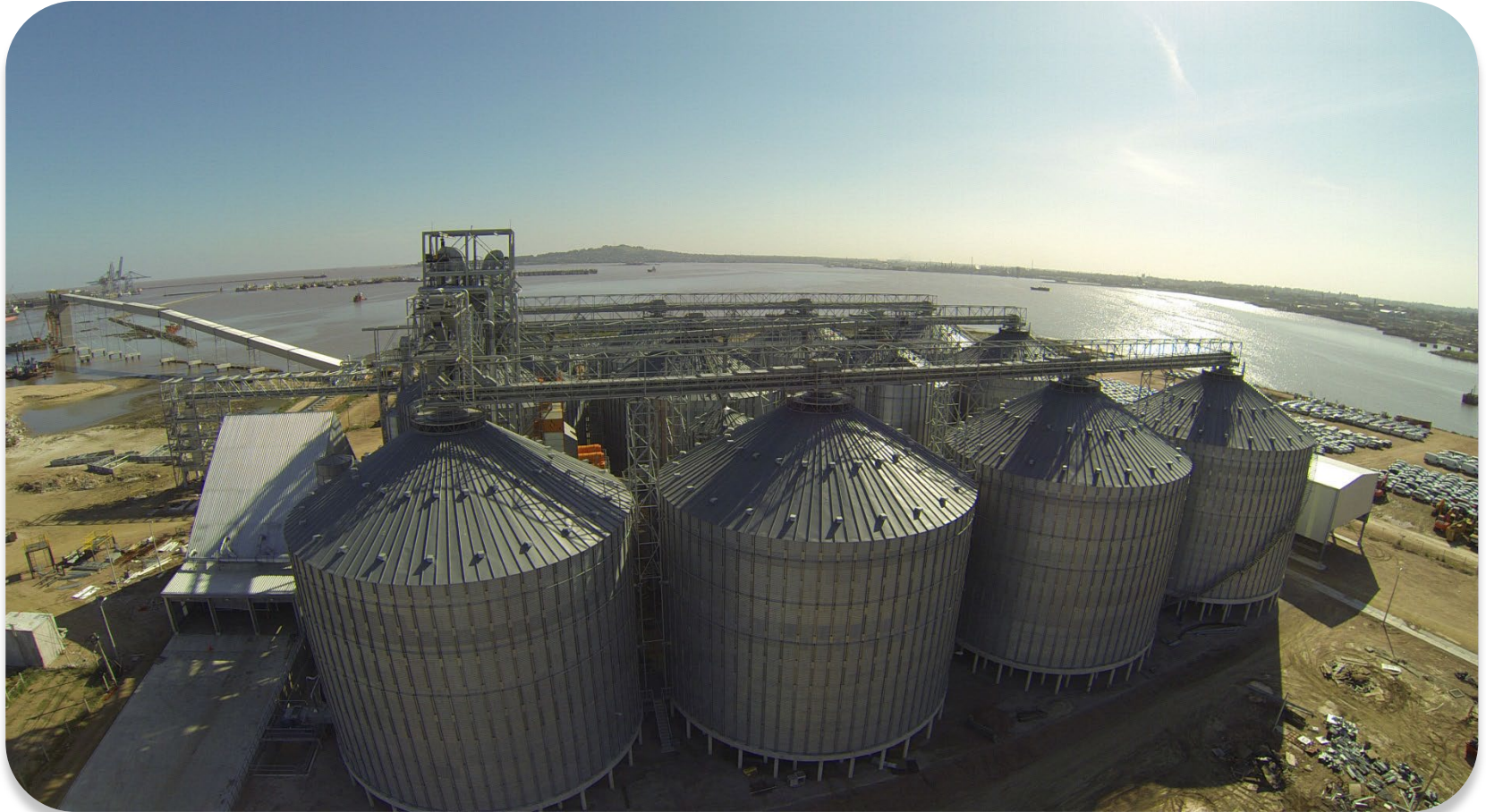
Silo installation with catwalks and catwalk towers
