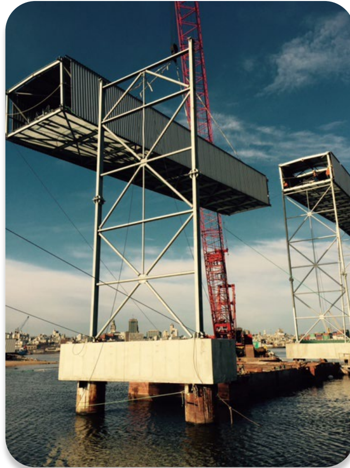
Tie-rod type structures for gallery support
