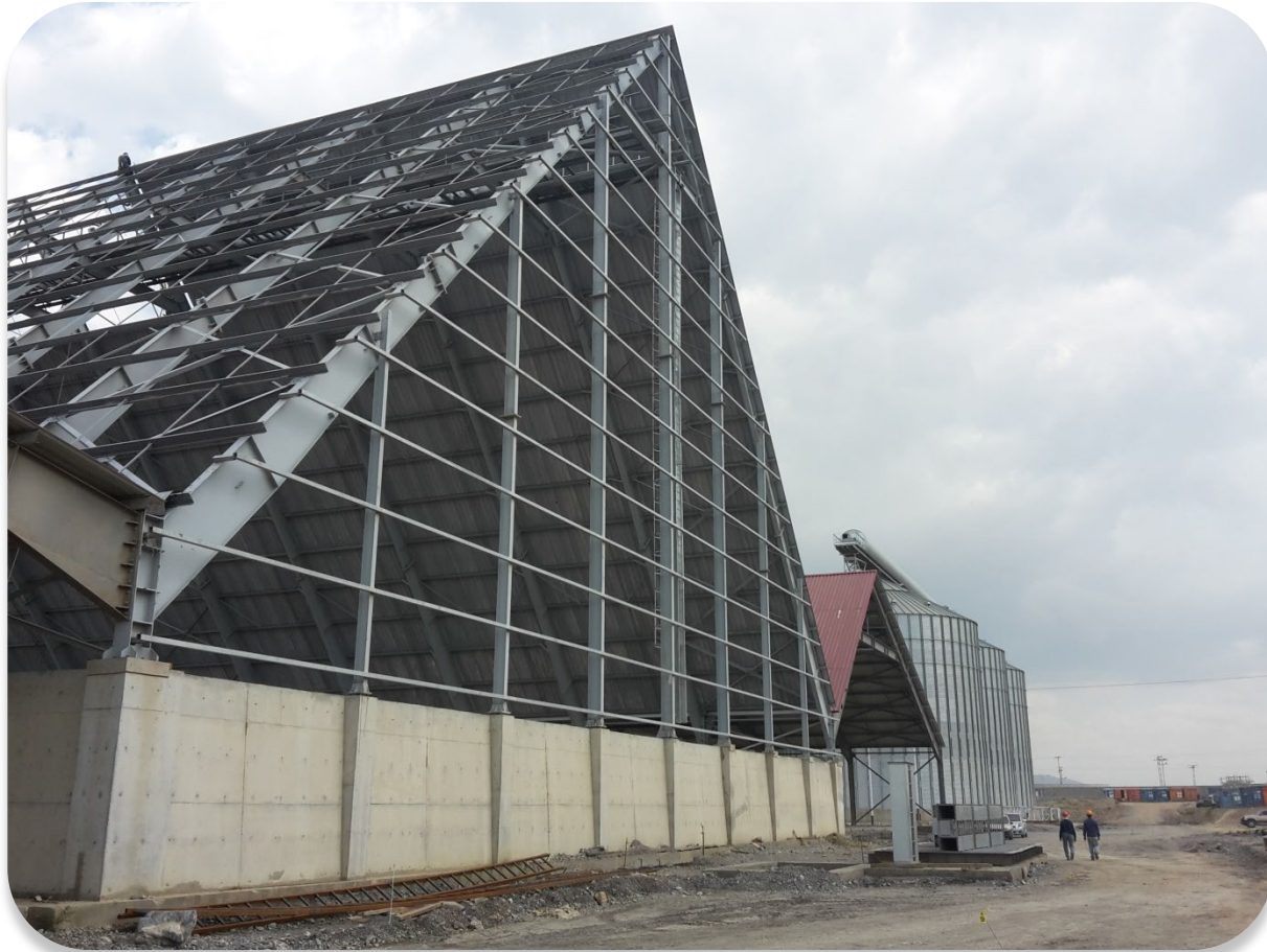
Bulk warehouse, h=45 m
