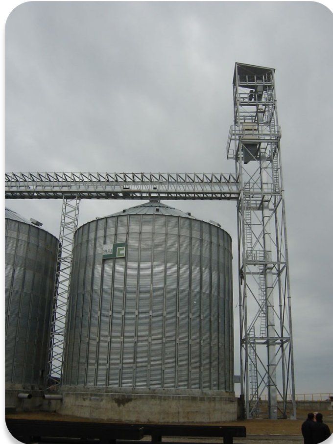
Intermediate tower, catwalk, and elevator tower
