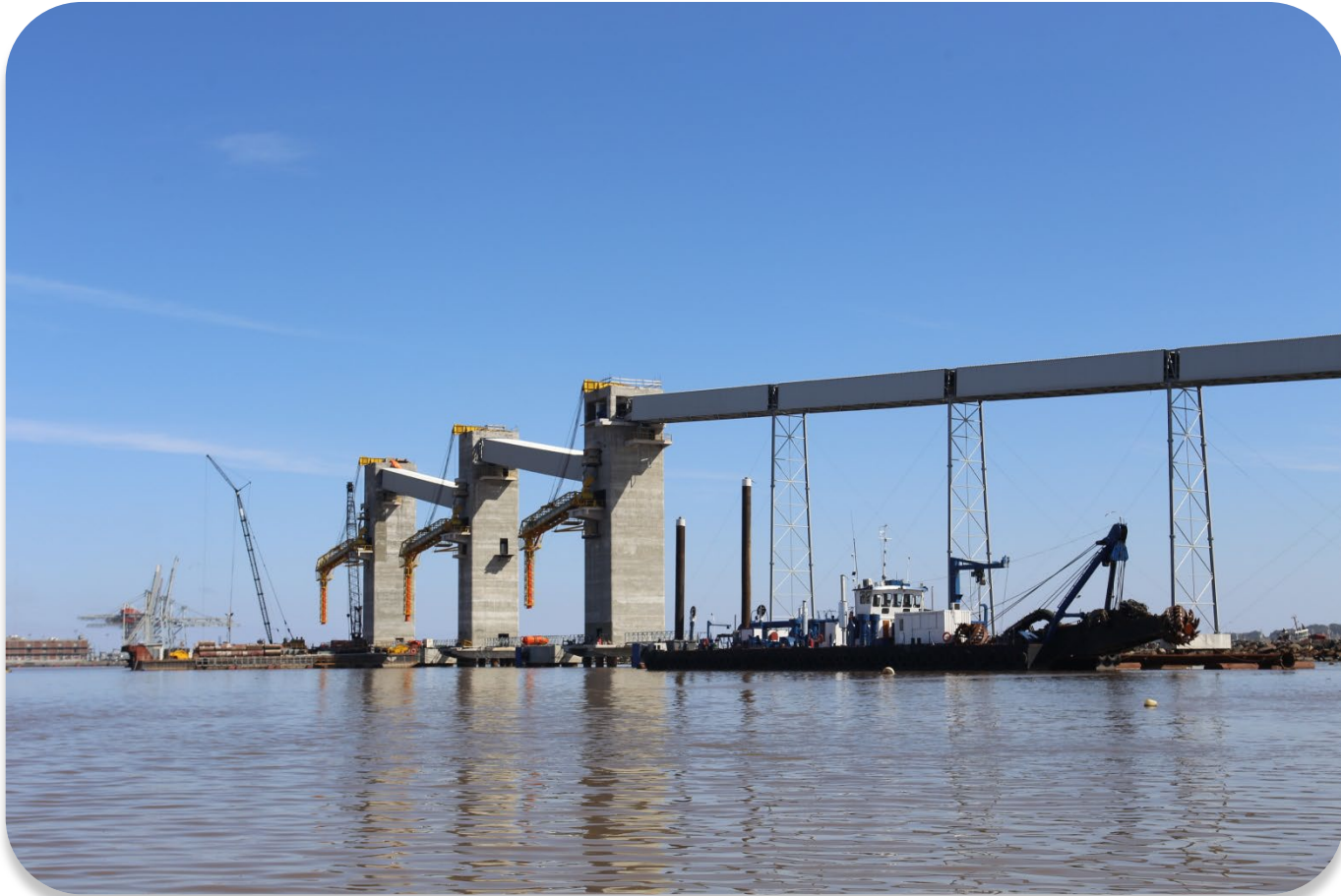
Tie-rod type structures for gallery support
