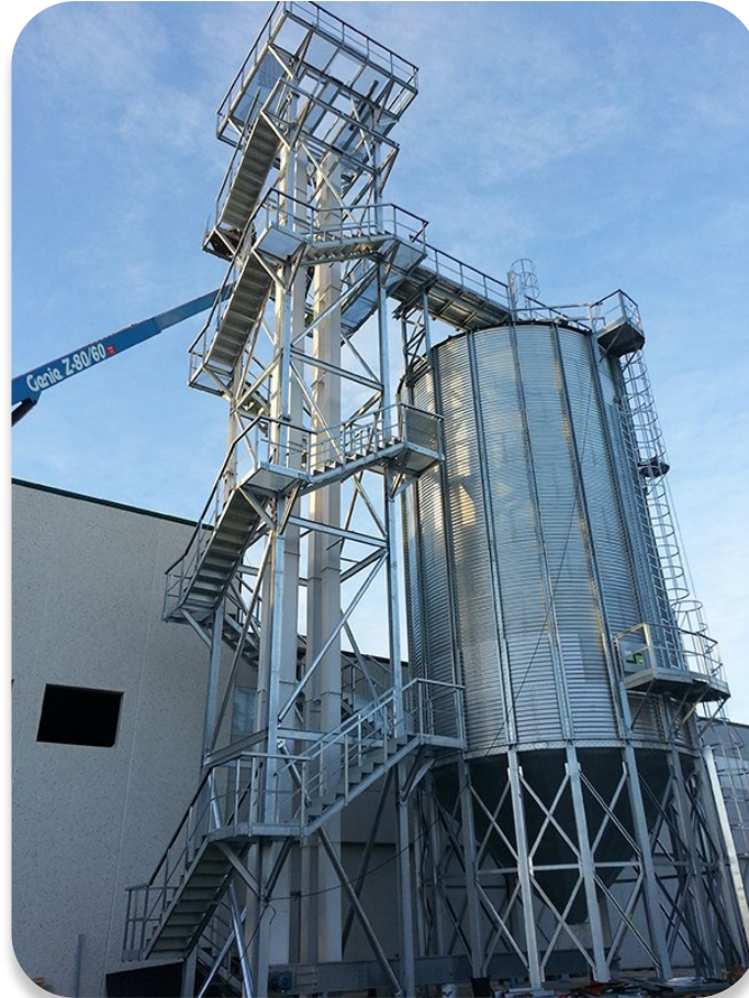
Access stair tower
