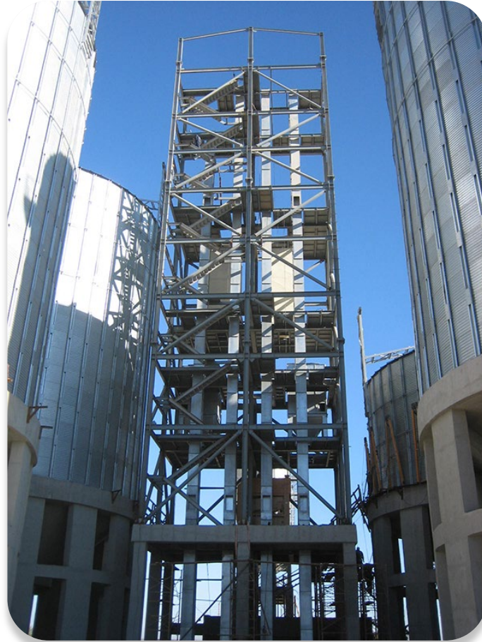
Elevator tower with access
