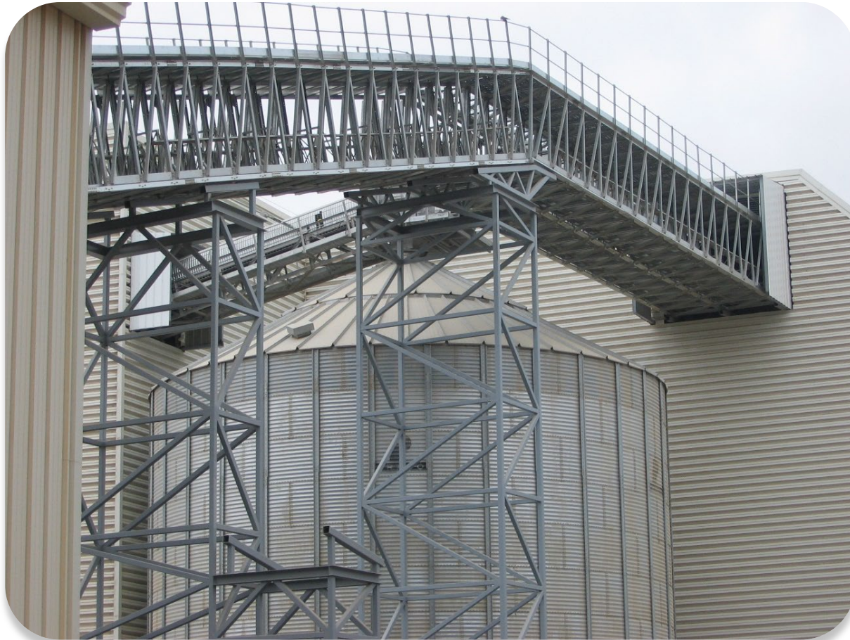
Support towers with catwalks
