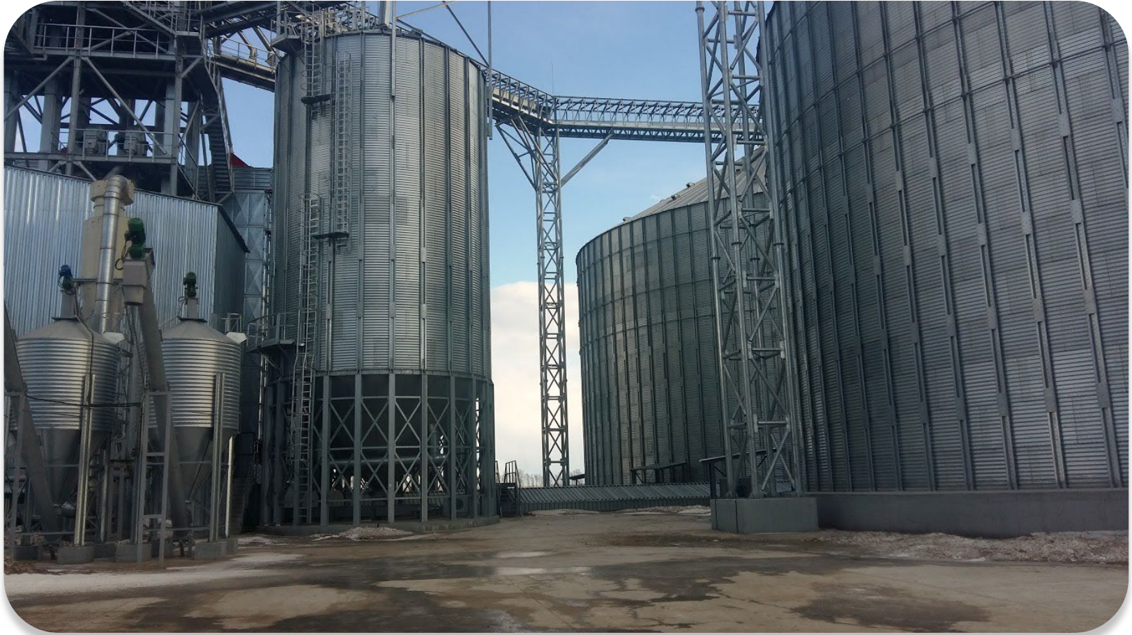
Silo installation with catwalks and catwalk towers
