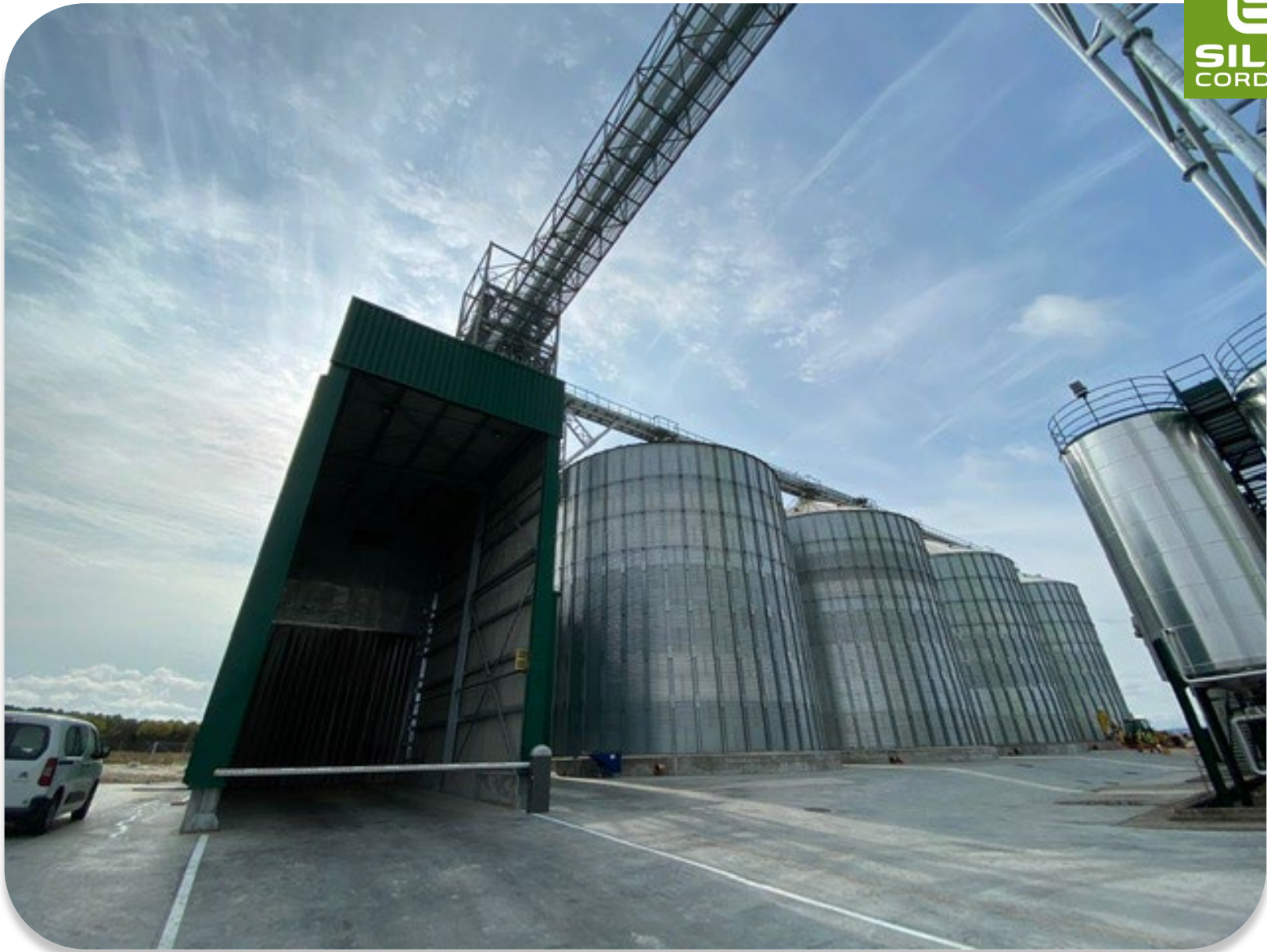
2020 ESAGROCE - SPAIN: 4 silos mod. 17,57/15 – Total Capacity: 14,250 T
