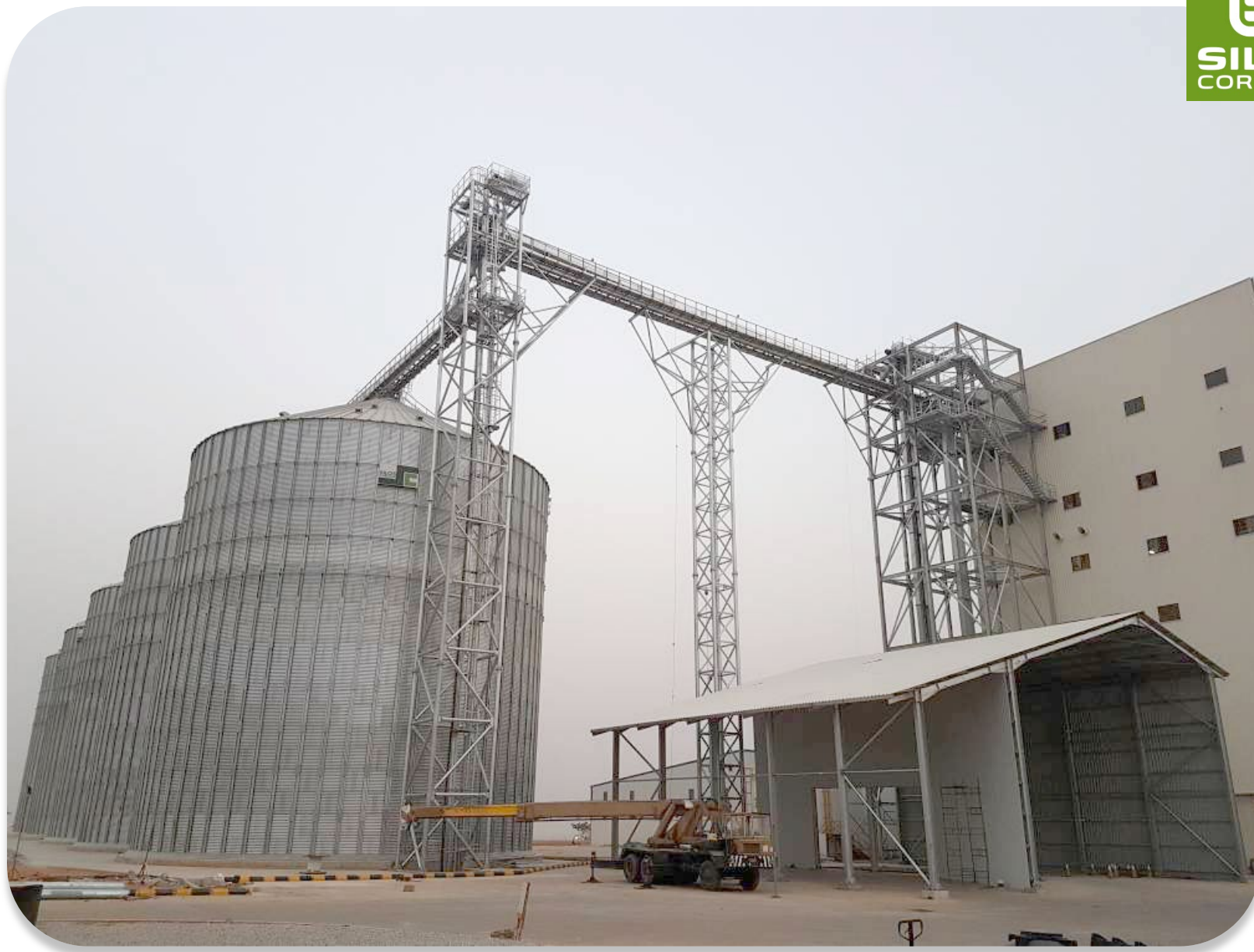
2017 NIGER04 - NIGERIA: 5 silos mod. 24,45/22 – Total capacity: 50.000 T
