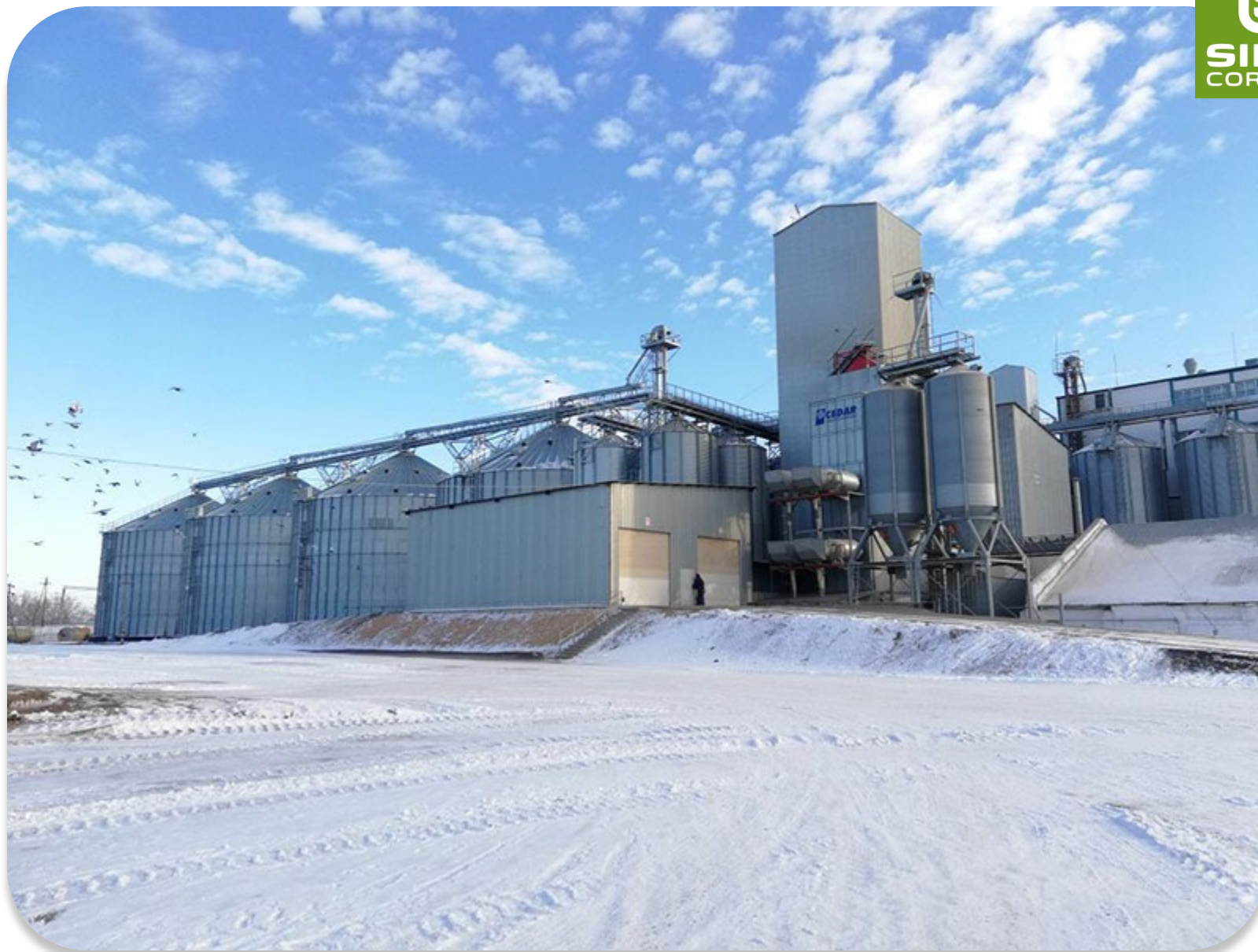
2019 TONKERIS – KAZAKHSTAN: 4 silos 17,57/13; 4 silos 22,92/13; 6 hopper silos 45° 5,35/9; 4 hopper silos 60° 7,64/10 – Total Capacity: 33,000 T
