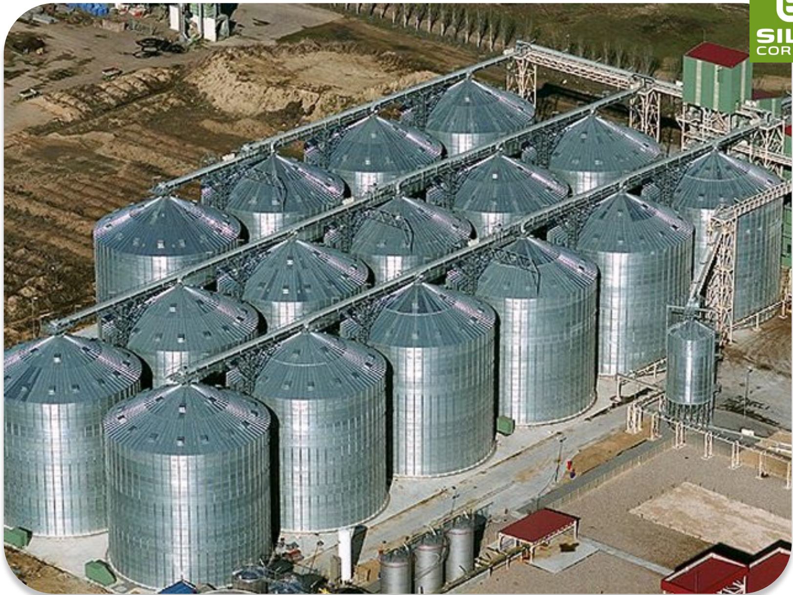
2007 ACOR- SPAIN: 16 silos mod. 27,50/22 – Total capacity: 200.000 T
