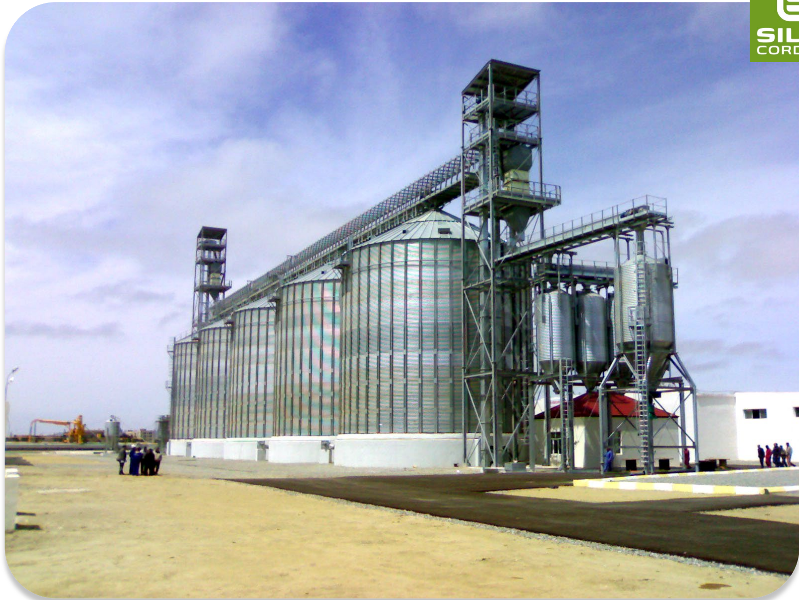
2007 BAKU – AZERBAIJAN: 5 silos mod. 16,81/14 – Total capacity: 15.000 T
