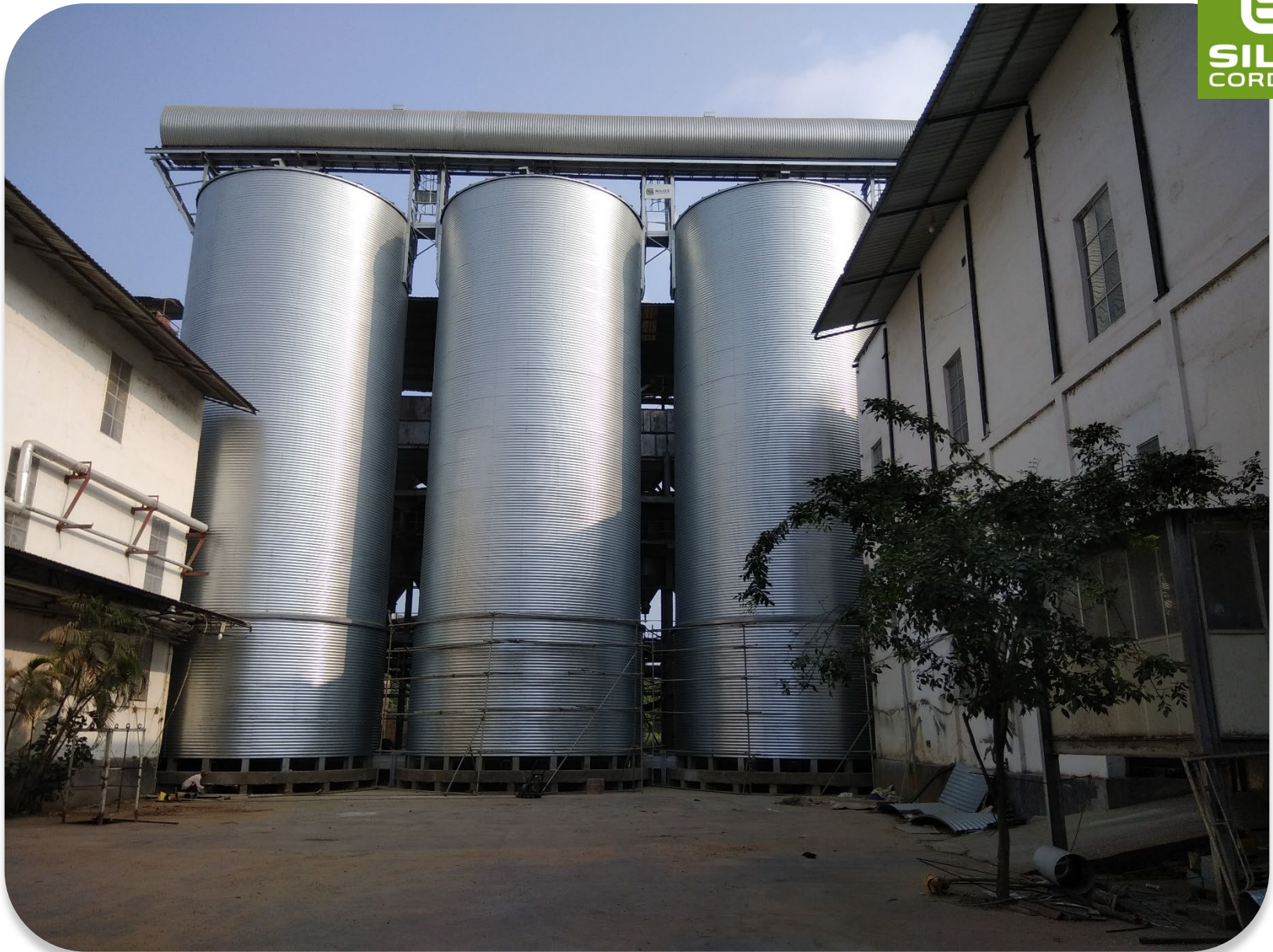
2019 SLK14 – SRI LANKA: 5 hopper silos mod. 10,70/8 45° – Total capacity: 4,000 T
