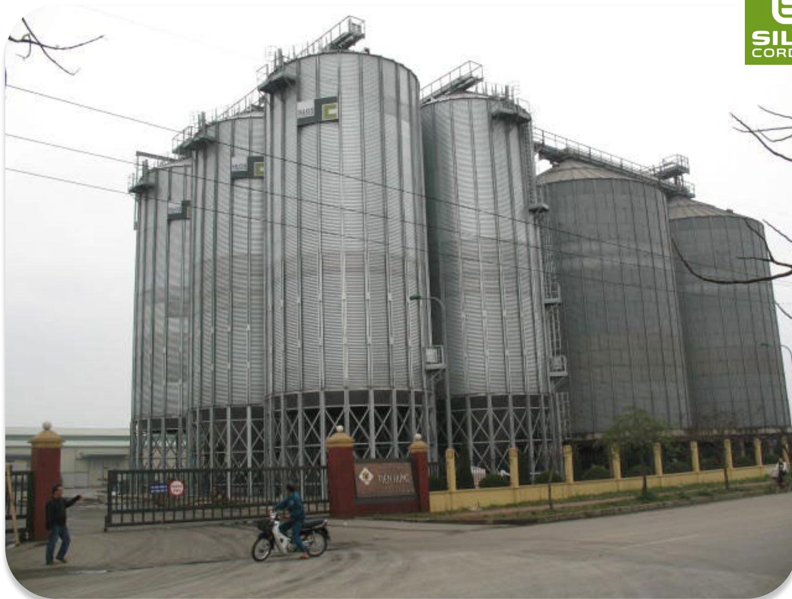
2008 TIEN HUNG - VIETNAM: 6 hopper silos mod. 9,17/16 – Total capacity: 6.900 T
