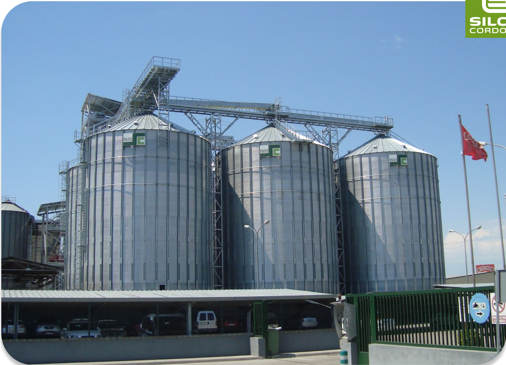
2013 ACEITES BORGES - SPAIN: 6 silos mod. 14,51/16- Total capacity: 14.600 T
