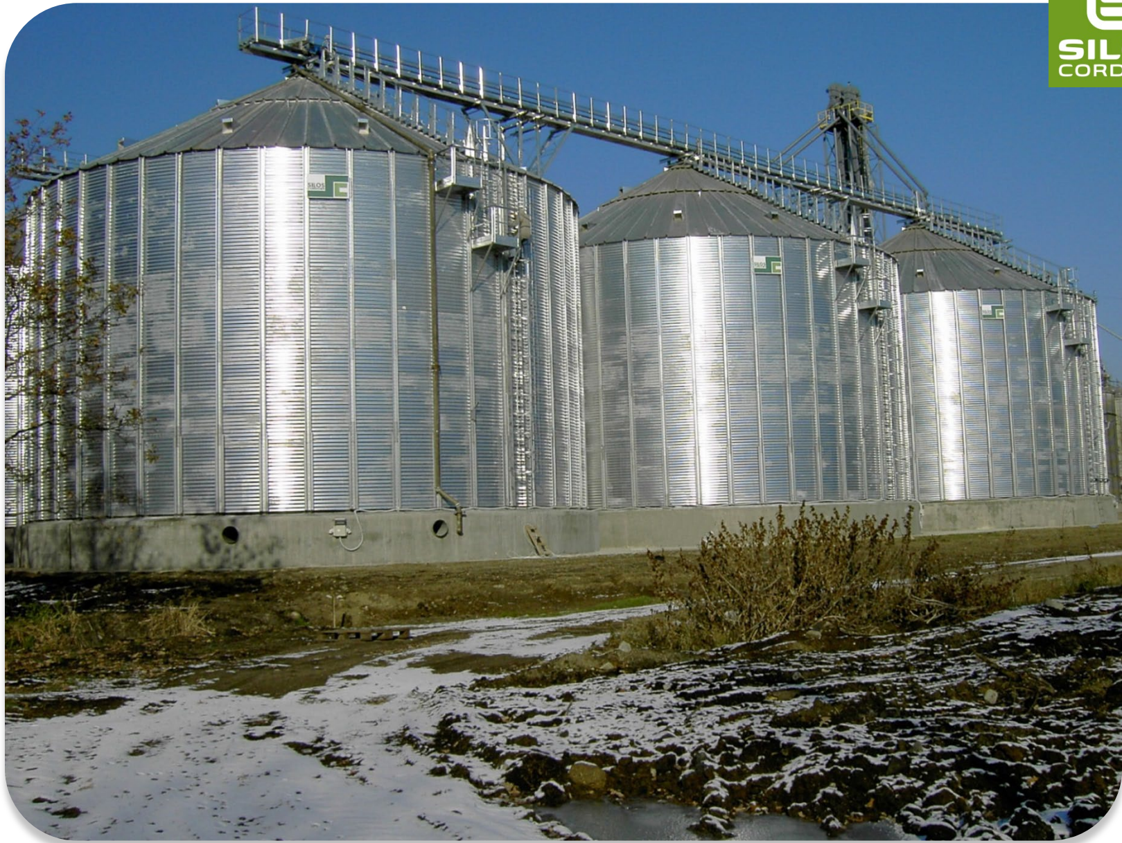
2005 HEVES - HUNGARY: 6 silos mod. 18,33/9 – Total capacity: 14.300 T
