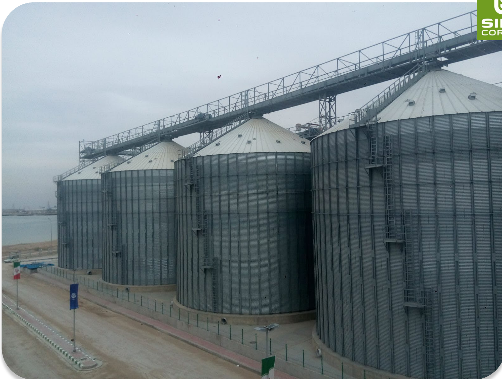
Under construction NKF - IRAN: 48 silos mod. 24,45/17 - Total capacity : 367.000 T
