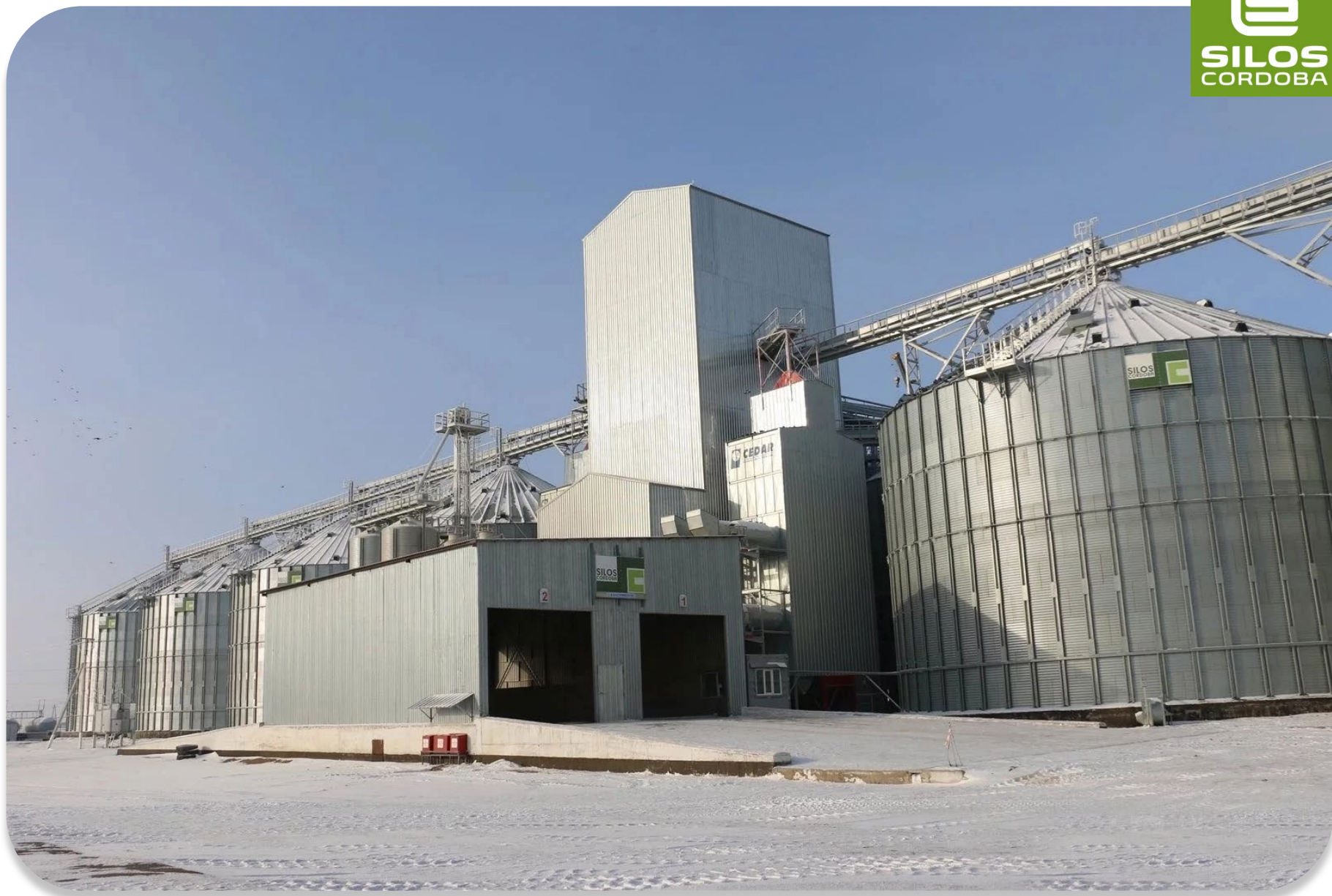
2017 IRCHENKO ELEVATOR - KAZAKHSTAN: 8 silos mod. 22,92/12 – 4 Hopper silos mod. 6,88/6 60° – 2 hopper silos mod. 6,11/9 60° – Total capacity: 40,750 T
