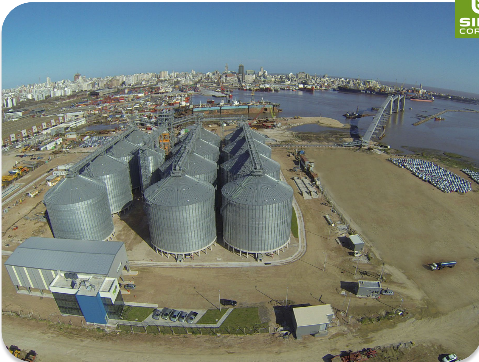
2015 OBRINEL - URUGUAY: 12 silos mod. 27,50/17 - Total capacity: 121.000 T
