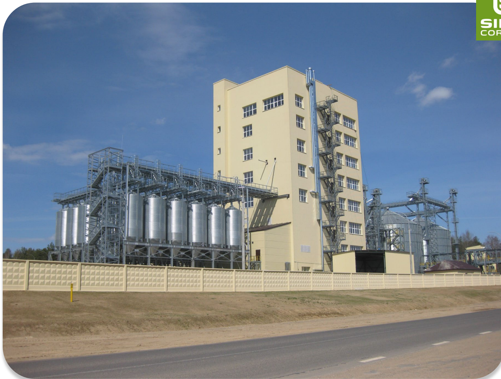
2015 VITEBSK - BELARUS: 8 silos mod. 19,10/13 – 14 hopper silos mod. 6,11/9 – 36 bulk load silos 3,50/5 - Total capacity: 33.800 T
