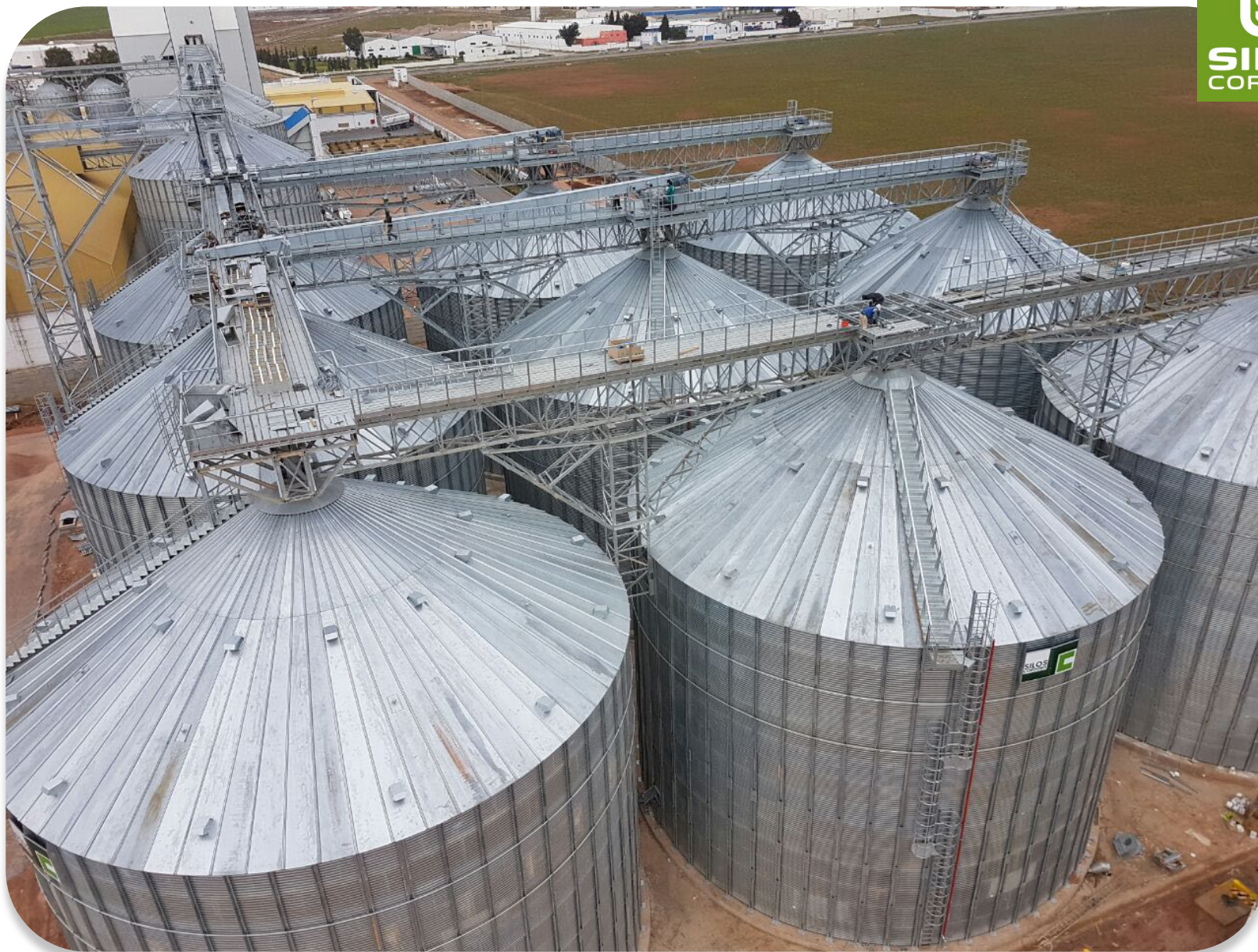
2016 SNA - TUNISIA: 10 silos mod. 22,92/14 - Total capacity: 56.400 T
