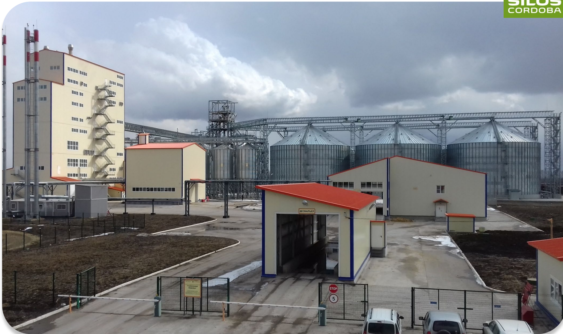
2016 INDEIKA - RUSSIA: 6 silos mod. 32,08/16 – 4 silos mod. 9,17/12 45° – 10 silos mod. 6,88/08 – Total capacity: 80.000 T
