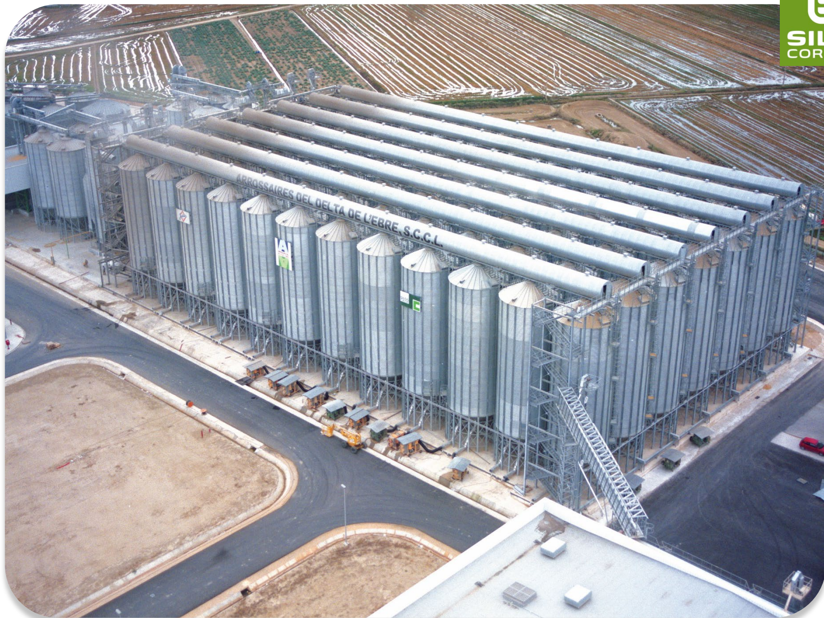
2004 ARROCERES DELTA DEL EBRO – SPAIN: 84 hopper silos mod. 7,64/16 – Total capacity: 69.000 T
