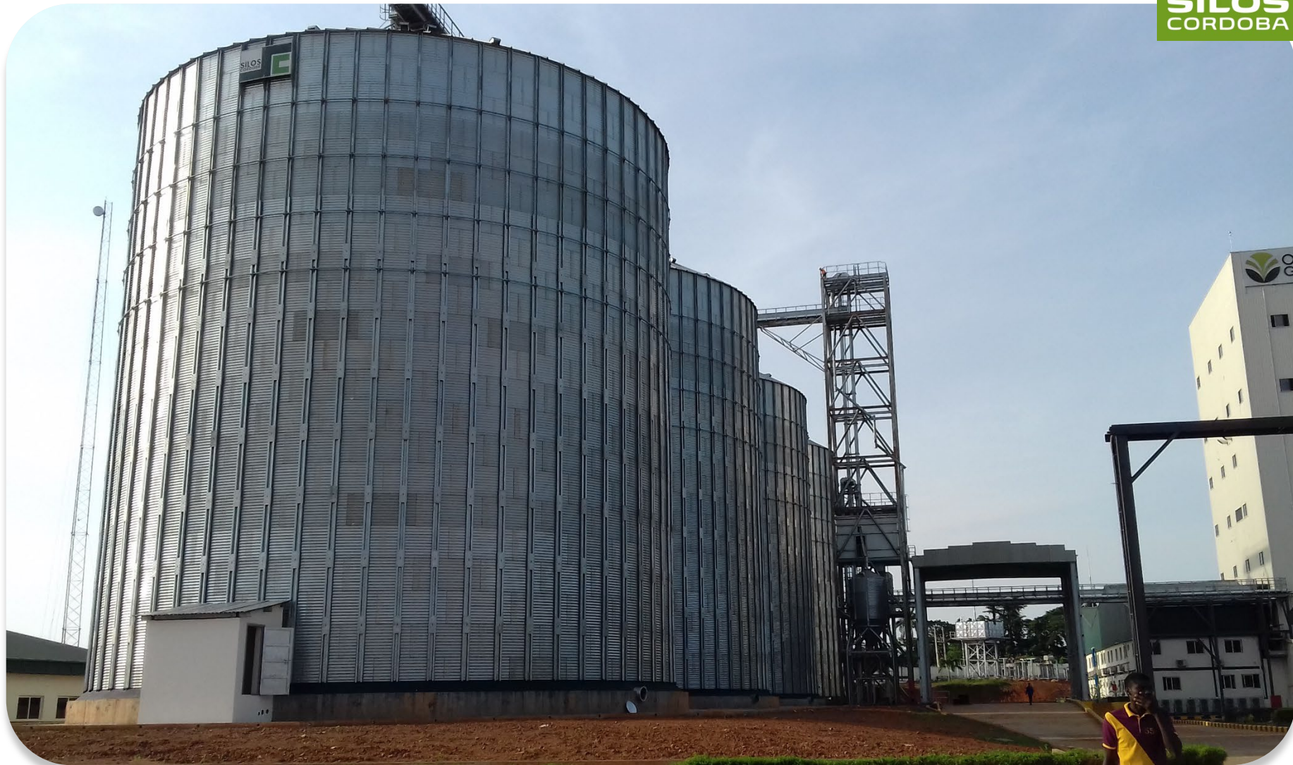
2017 NIGER05 - NIGERIA: 4 silos mod. 24,45/22 – Total capacity: 40.000 T
