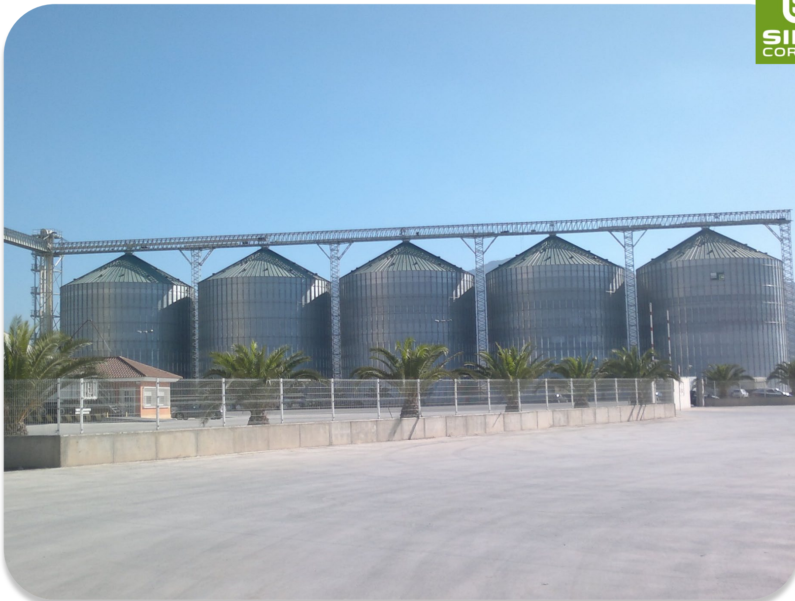
2011 CEFUSA – SPAIN: 5 silos mod. 27,50/22 – Total capacity: 62.000 T
