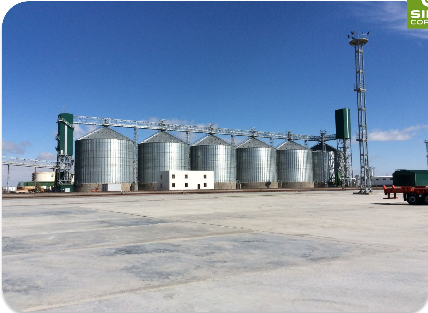
2015 AKT - KAZAKHSTAN: 6 silos mod. 27,50/18 - Total capacity: 62.000 T
